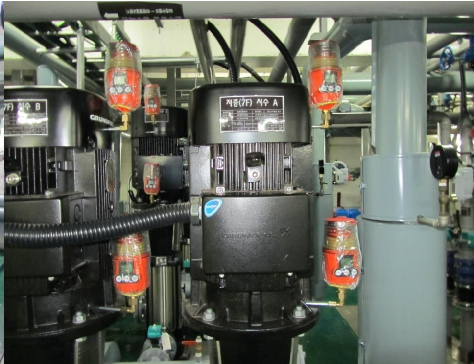
Pulsarlube M installed at vertical water pumps in HVAC systems of local hotel.
