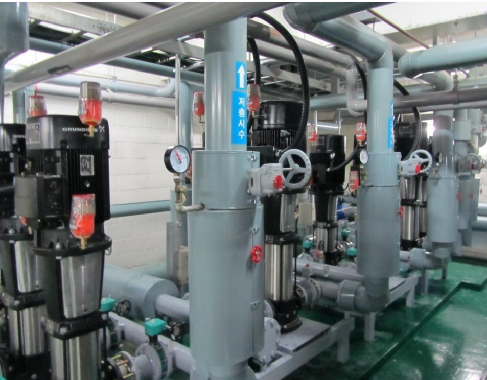
Pulsarlube M installed at vertical water pumps in HVAC systems of local hotel.
